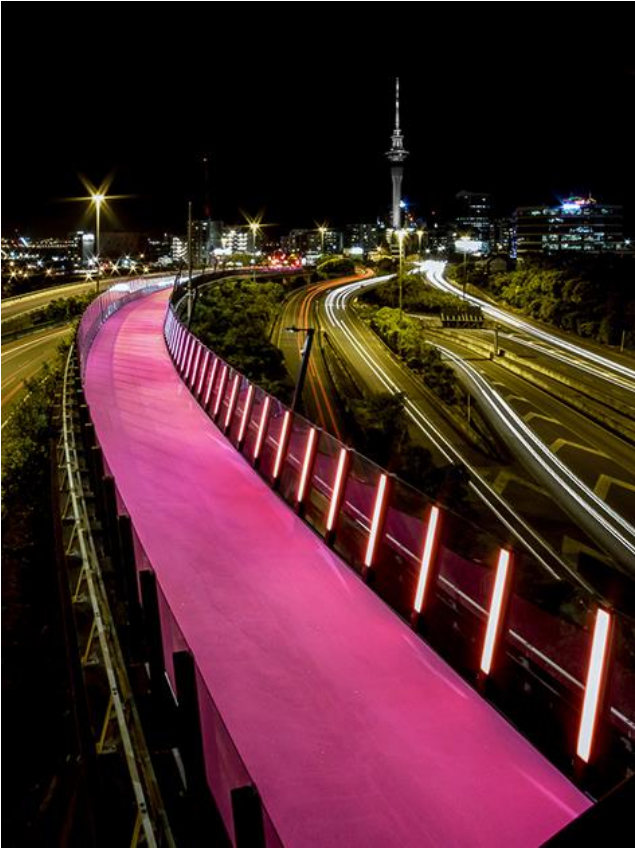
Nelson Street Cycleway (Toronto) Statement route through the city
